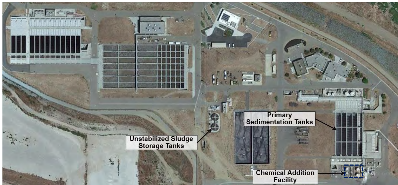
Figure 7-14. Chemical Addition Facility and Dosing Locations.
